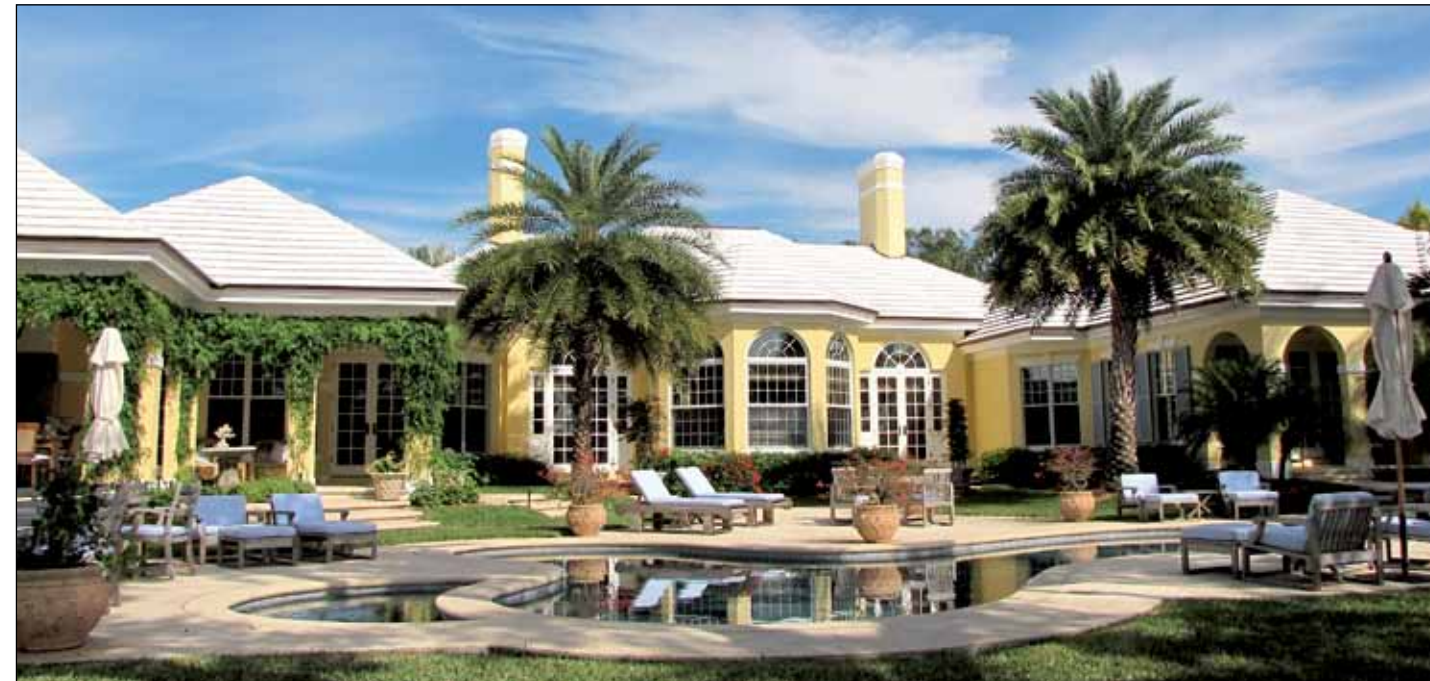
An example of the exquisite estates on Gem Island – this one not for sale – where the community's traditional Georgian architecture is taken to the extent of its creative potential by talented architects.
